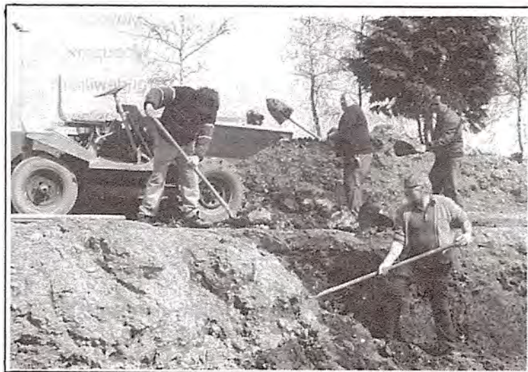
Digging the deep foundations for the slipway walls.
